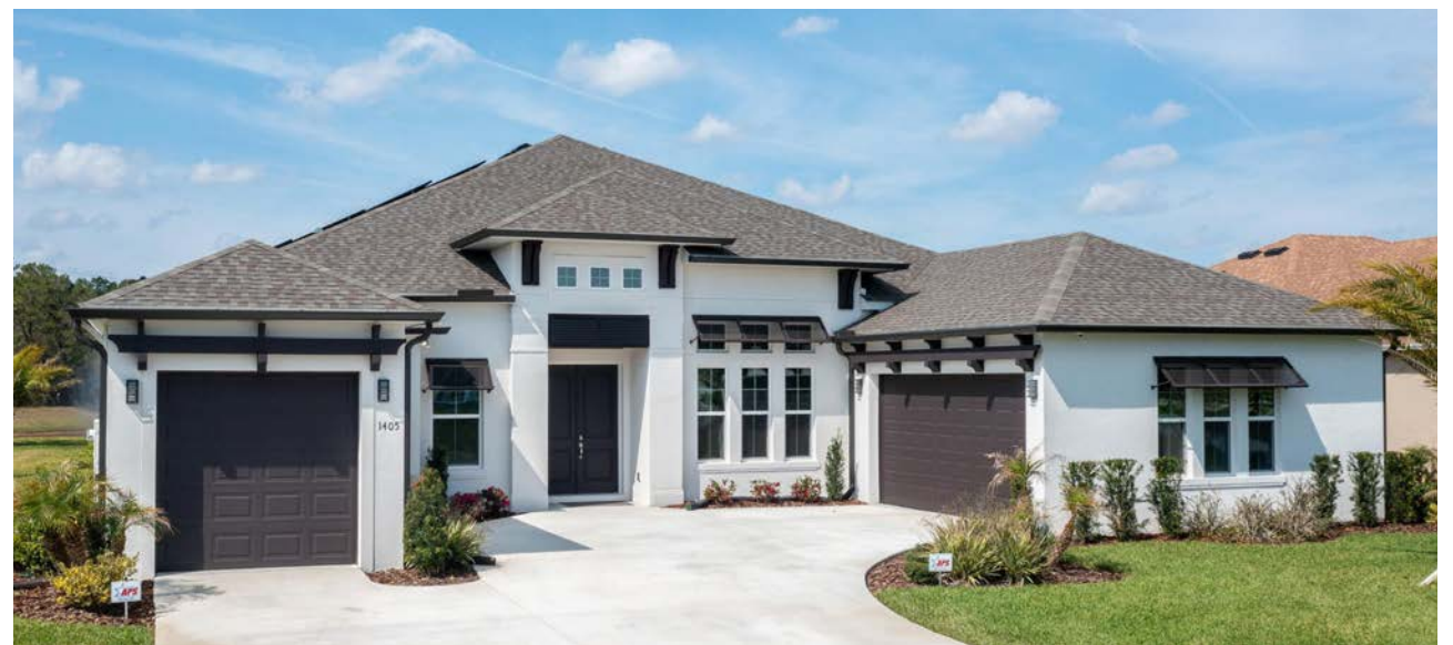
The house at 1405 Lilly Anne Lane has 3,270 square feet of living space.
