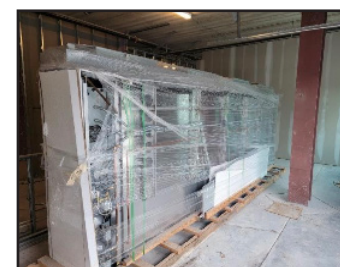
The exhaust hood is large and heavy, measuring over 30 feet long and weighing hundreds of pounds.
